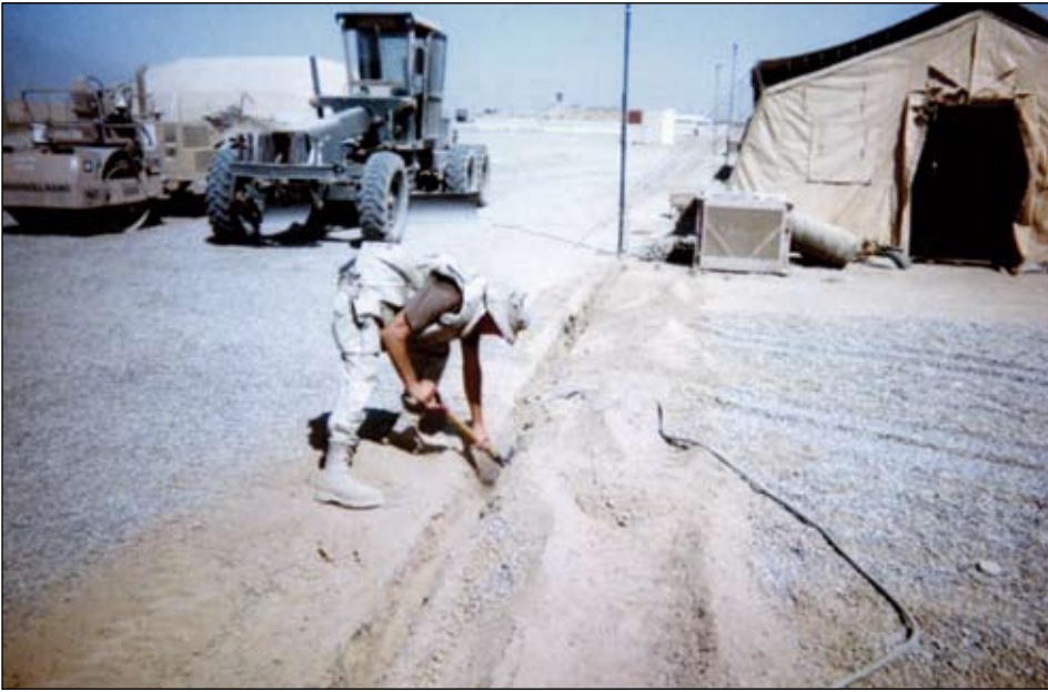
Master Sgt. Greg Sielepkowski digs a trench for an electric line in Tent City at Kirkuk, Iraq.
