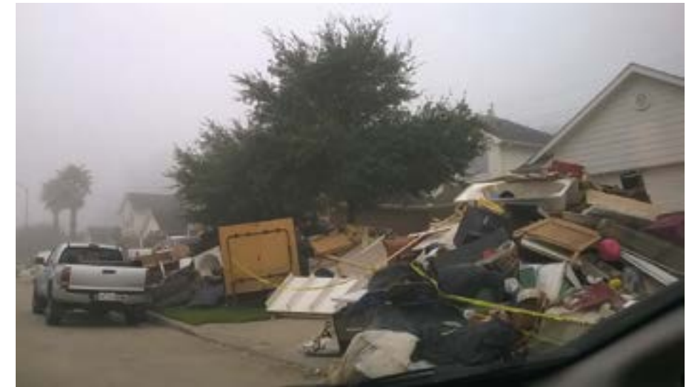
Some houses were so badly damaged the first step in restoration was gutting them.
