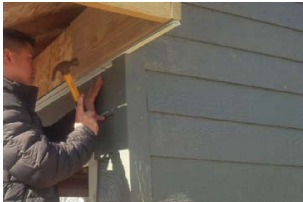
Lopez nails a piece of siding in place.
