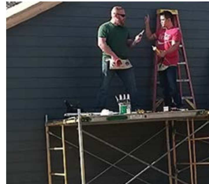
Jordan Gray and Lopez consult while siding the garage.
