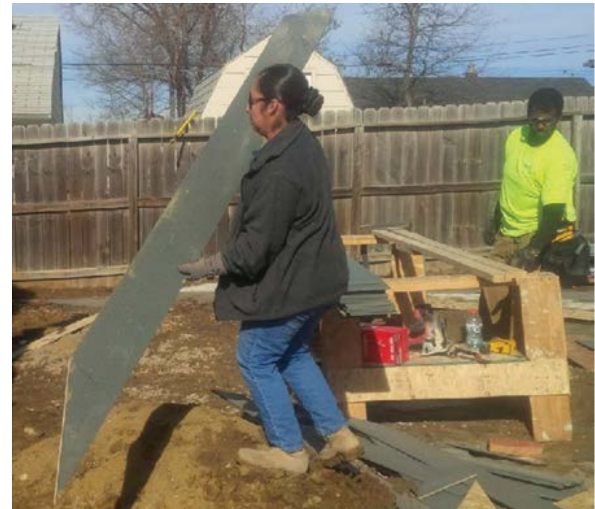
1st Sgt. Zulma Gray delivers a piece of siding.
